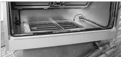
Fig. 33: Extract air filter installed in the unit
