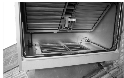
Fig. 43: Extract air filter
