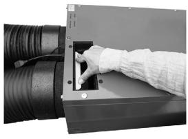
7. Insert prefilter cover and lock it with the latches
