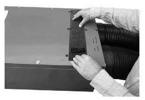
8. Lock the filter cover with the six latches
