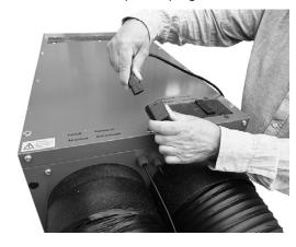
2. Place screwdriver and pull out insert
